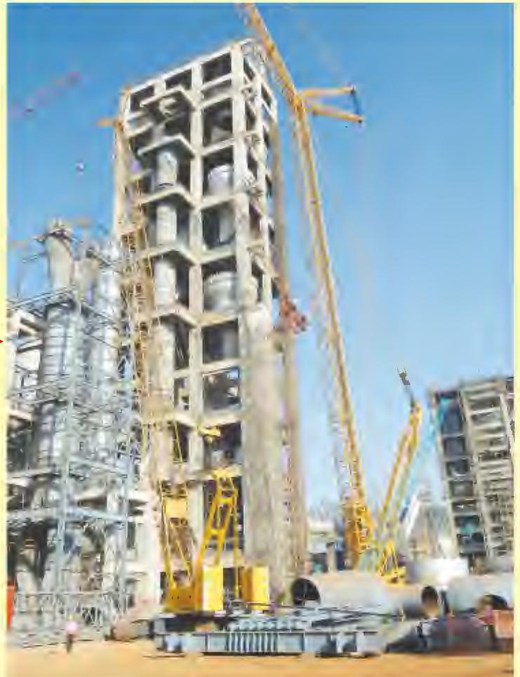
LIEBHERR LR1750 (Capacity 750MT) Crawler Crane, Erection of PRE-HEATER CYCLONE at Height - 168m Crane Configuration SDWB 91m + 105m at ACC Limited, Chhattisgarh.
