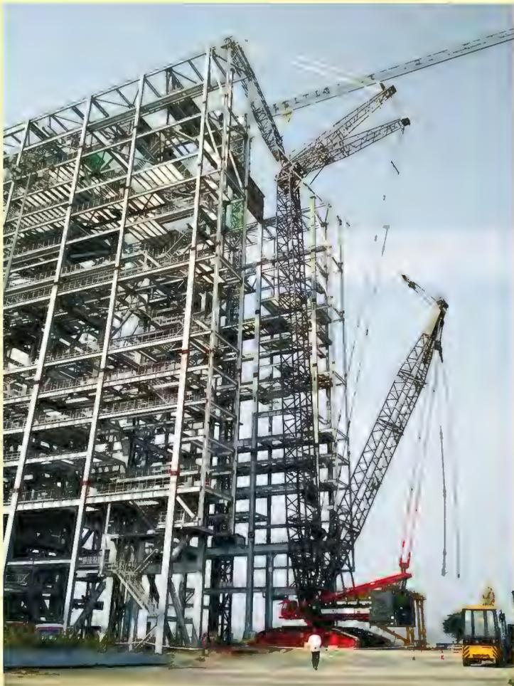
LIEBHERR LR1800 (Capacity 800MT) Crawler Crane, Erection of CEILING GIRDER of Weight – 212MT at Height – 90m with Crane Configuration SDW 70m + 42m for 2 x 660MW Lanco Vidarbha Thermal Power Project, Wardha, Maharashtra.
